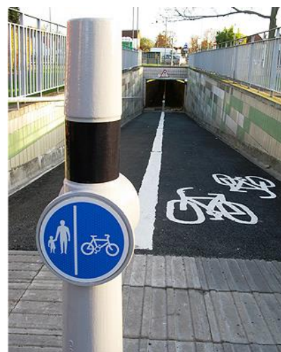
Photo 28 - Example of TSRGD 957 on Bollard
