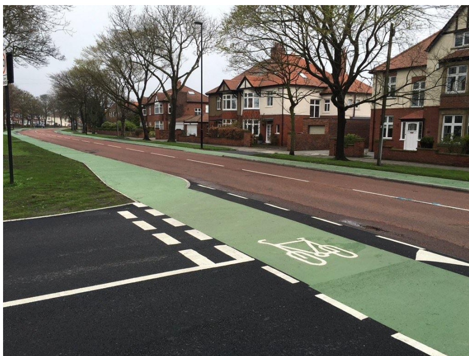
Photo 19 - Example of raised table at priority junction at The Broadway, Tynemouth
