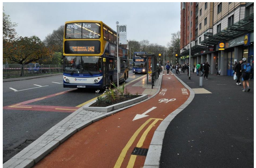
Photo 9 - Example of Bus Stop Bypass in Manchester
