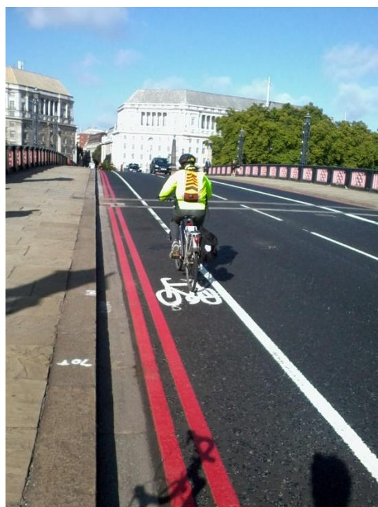
Photo 6 - Example of mandatory cycle lane in North London, these are represented by a continuous line that should not be crossed
