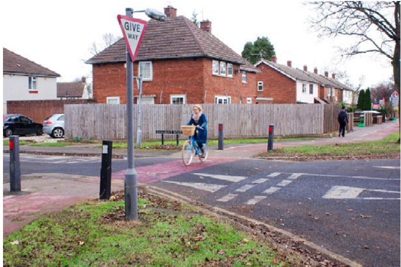
Photo 2 - Level surface priority crossing on side roads (Making Space for Cycling)
