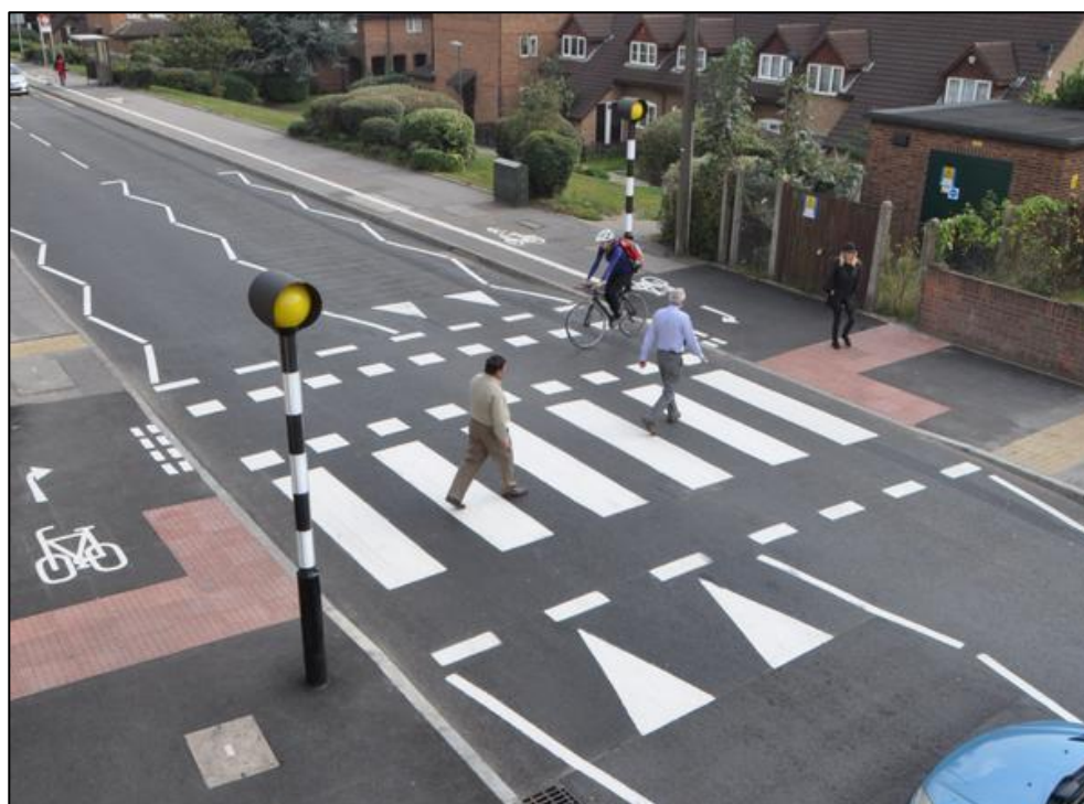
Photo 26 - Example of Parallel Crossing in Bexley, London
