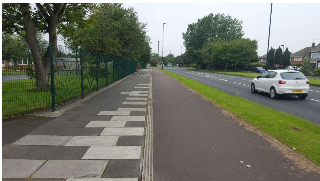
Photo 3 – Footway and Cycle Track on Beach Road, Tynemouth, clearly distinguished by surface treatment
