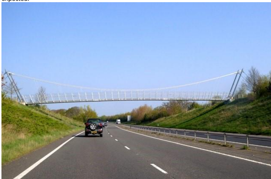
Photo 29 - Example of Footbridge over A5 near Nesscliffe Hill
