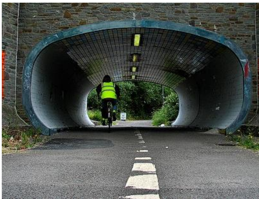
Photo 28 - Example of underbridge in Bristol
