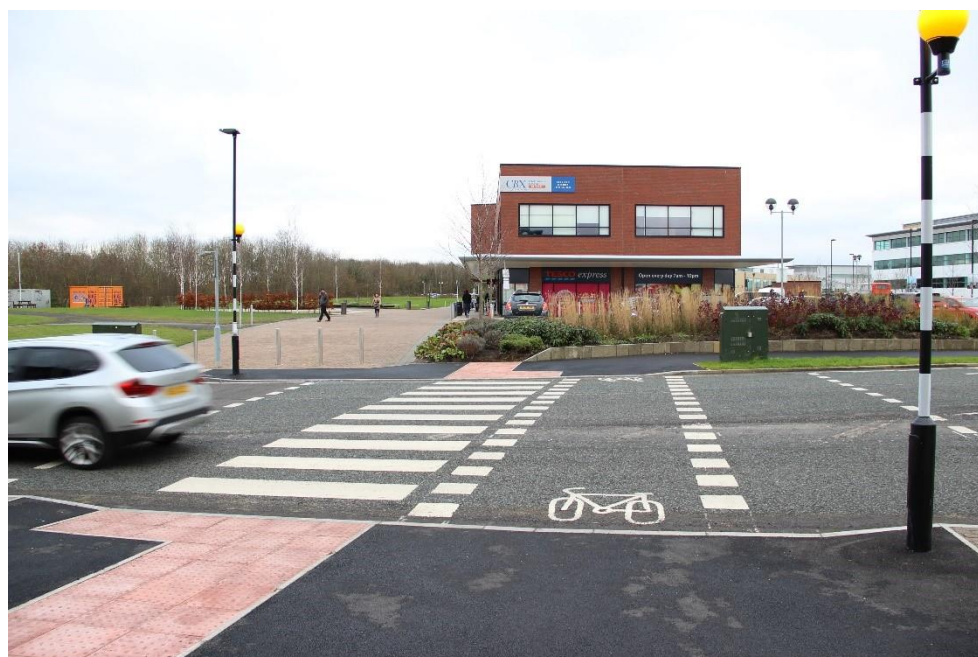
Photo 30 - Example of Parallel Crossing in North Tyneside
