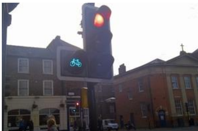
Photo 21 - Example of an early release traffic signals head
