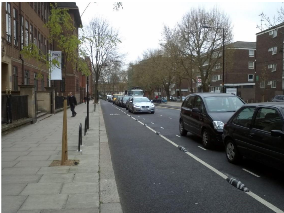
Photo 5 - Example of light segregation using armadillos (Royal College Street, London) – note inclusion of car door zone
