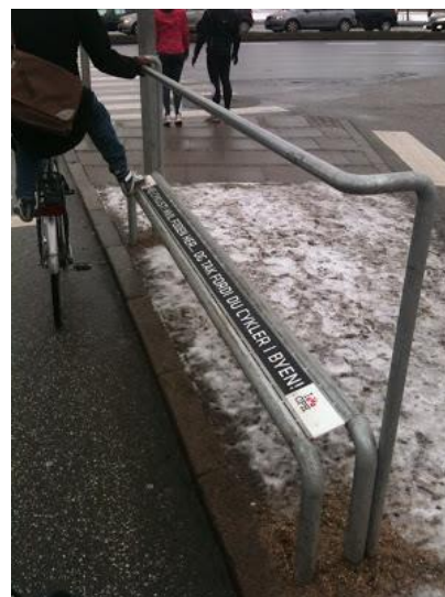
Photo 22 - Example of railing / footrest
