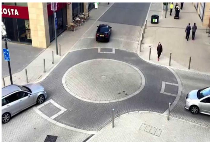
Photo 27 - Example of Informal Roundabout
