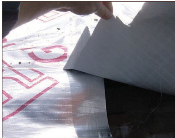
Figure A4.76 No double sided tape used in joints (courtesy Smith Grant)
