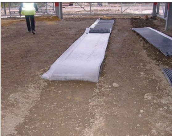
Figure A4.35 Good installation of passive gas venting trenches and 'egg-crate' (courtesy Card Geotechnics Limited)
