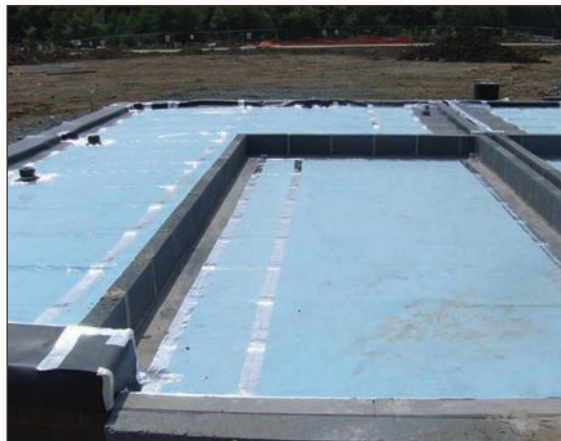
Figure A4.10 Almost complete coverage available for inspection, minimal jointing, service entries suitable distance from walls, light traffic (courtesy Smith Grant)
