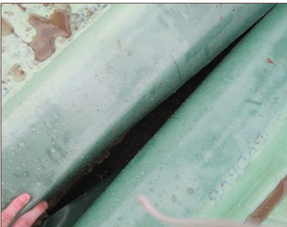
Figure A4.59 Gas membrane slit at the bottom of a cavity tray to enable water to drain away (courtesy Smith Grant)
