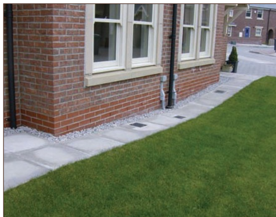
Figure A4.36 Raised air bricks are preferable due to the reduced potential for blockade but the vent trench specified is provided with clean single sized stone (courtesy Smith Grant)
