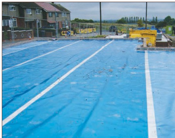
Figure A4.60 Some stones could penetrate gas membrane if sufficient force is applied (courtesy Smith Grant)
