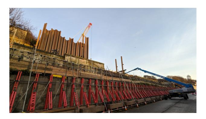
We have now completed the slope stabilisation works with the last piling completed week beginning 5 February. The large crane on Tyne Street used to do the piling works has been dismantled and removed from site.
