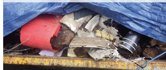
Top: The former plant room with asbestos debris on the pipes and floor. Bottom: Asbestos was left in an open skip.
