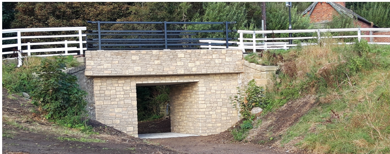
Pier Road Bridge
