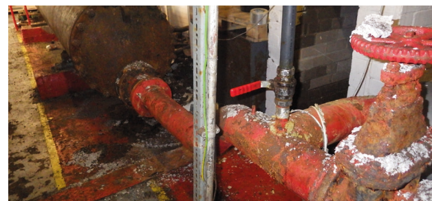
Top: The former plant room with asbestos debris on the pipes and floor. Bottom: Asbestos was left in an open skip.
