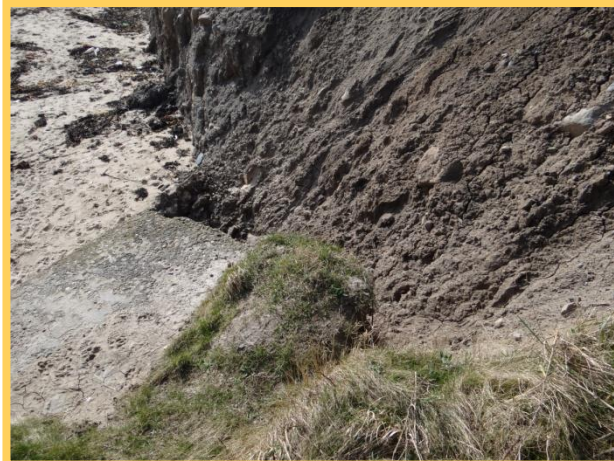
Figure 2-5 Erosion outflanking Trinity Road seawall
