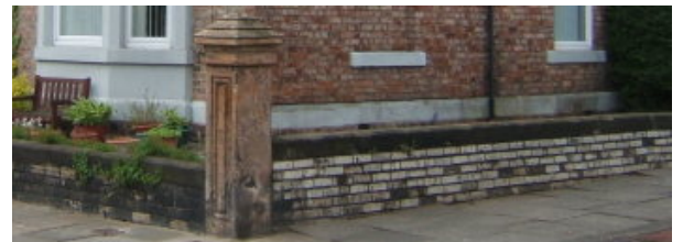
Boundary walls with stone plinths on salt-glazed bricks, and gate pier
