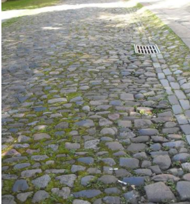
Historic road and pavement surface, Camp Terrace
