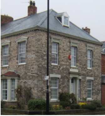
Hipped roof, Waterloo Place/Fenwick Terrace
