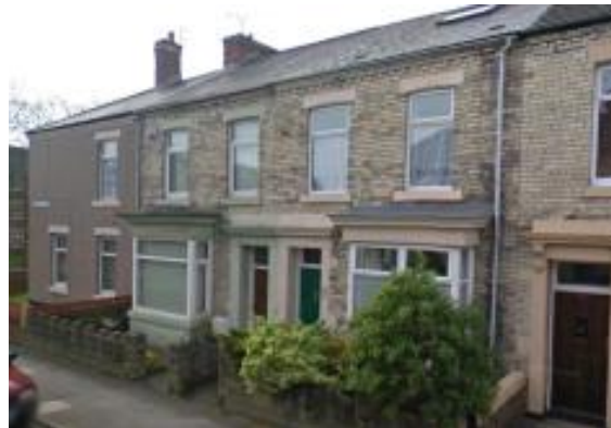
Pebbledashing concealing historic brickwork
