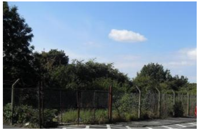
Rich, mature tree coverage but poor quality boundary treatment
