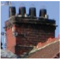
More square chimney on Edwardian property
