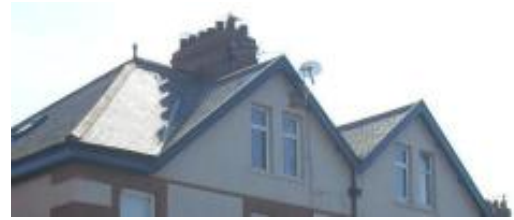
Welsh slate roof with terracotta ridge tiles and finials, Cleveland Crescent
