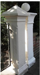
Gate piers, Alma Place
