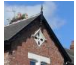
Verge with moulded timber bargeboard and finial, Alma Place
