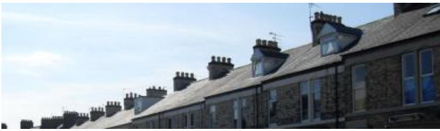
Chimneys creating a lively roofscape, Alma Place
