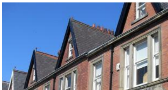
Gables, nos.7-12 Camp Terrace
