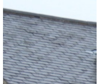
Welsh slate roofs with grey interlocking ridge tiles
