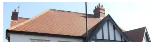
Red clay plain tiled roof, Cleveland Crescent
