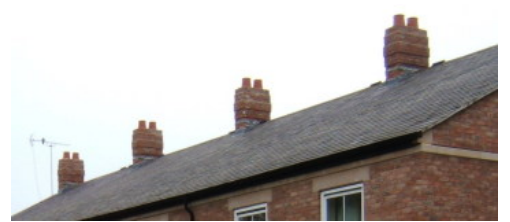
Smaller chimneys on newer properties
