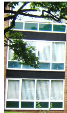
Green panels add interest at Etal Court
