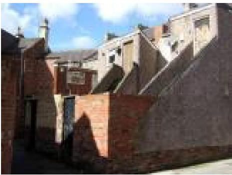
Even on tight corner plots, each house or flat has a rear access or yard squeezed into the layout
