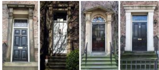
Typical original and high quality replacement doorways
