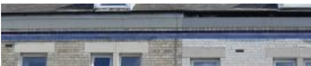
Coloured salt-glazed bricks, Alma Place
