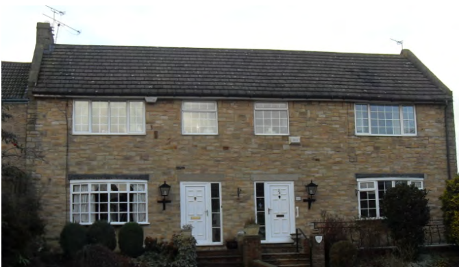
Two-storey, pitched roof buildings are common in the village
