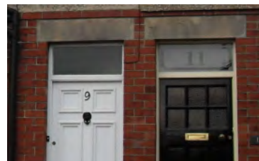
Simple stone lintel and overlight
