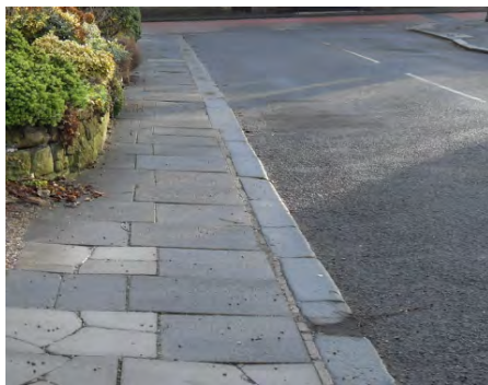
Modern surfaces with historic granite kerb
