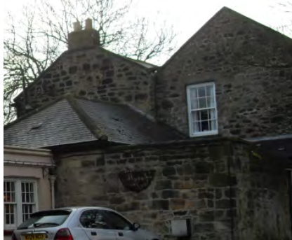
Double pile roof
