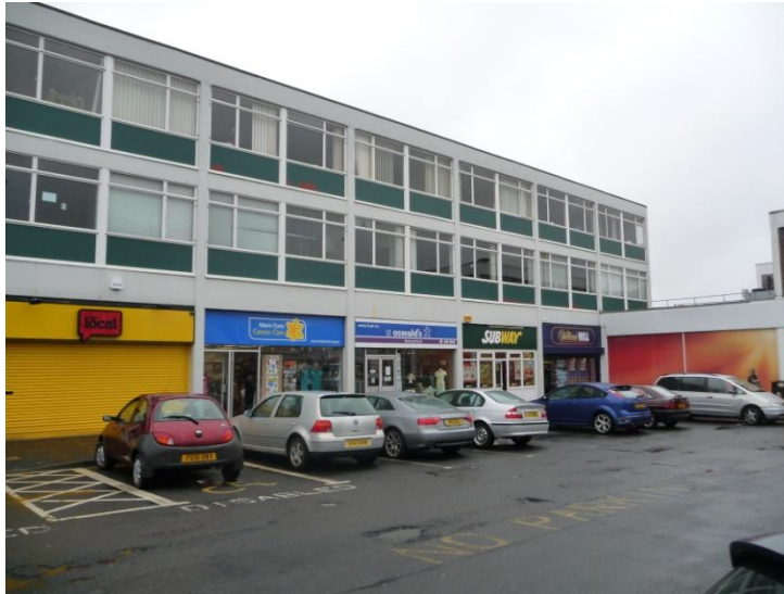
Figure 5 Car parking in Forest Hall and low architectural quality of building
