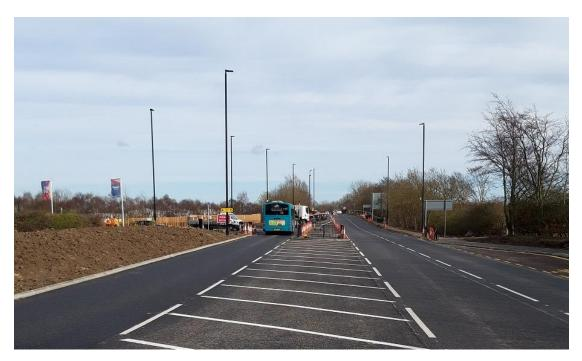
On the southern side of the road, the team has completed the bus lay-by as well as installed the lighting columns and infrastructure for the new traffic signals. However, the lights will not be in operation until adjustments are made to Weetslade roundabout later this year.
