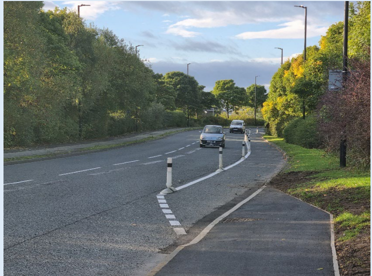
The new segregated cycling facilities on Middle Engine Lane
