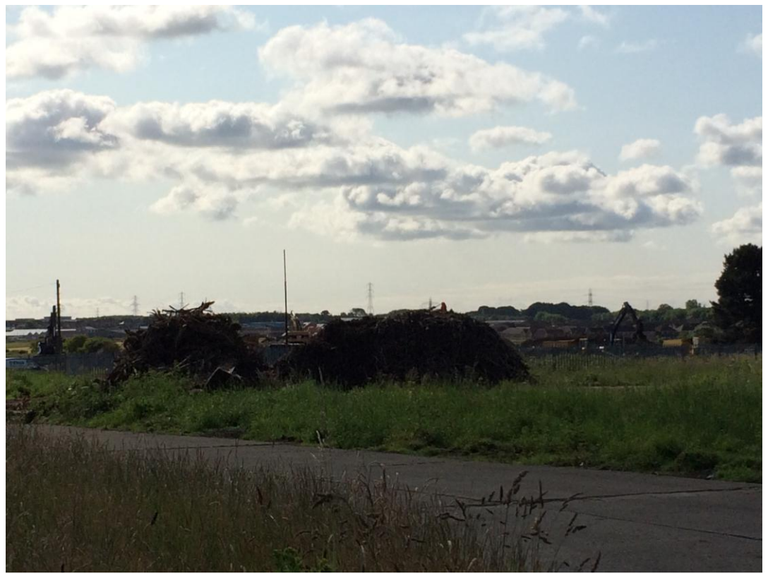
Plate 9. Stockpiles of demolition material on the site of the former depot.
