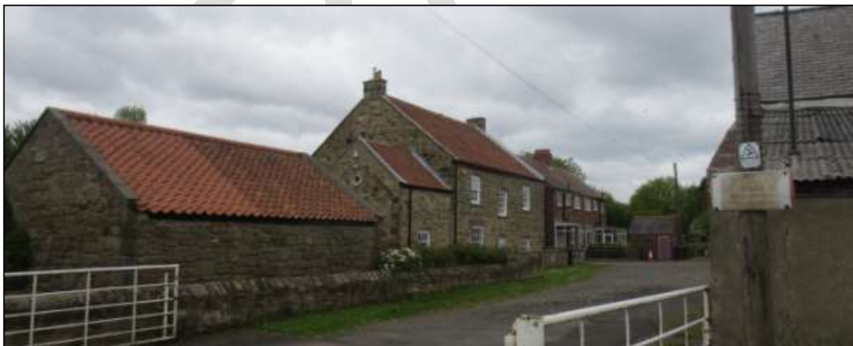
Figure 15: East House Farmhouse’s rear and eastern elevation, seen from the road
