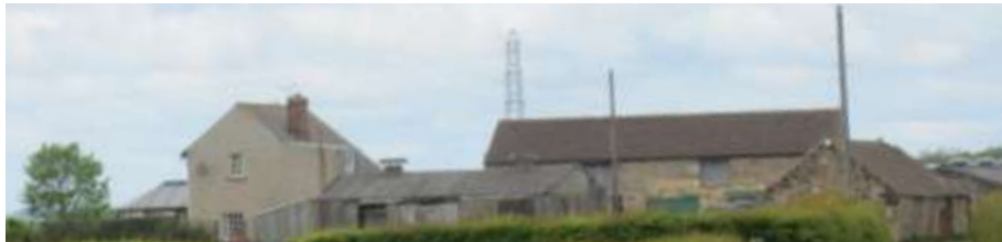
Figure 05: Holystone Farm from the east with older barns surrounded by more modern development
