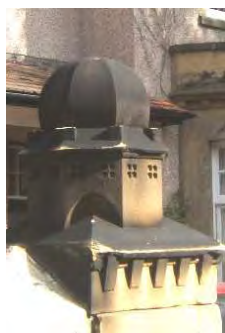
Unusual pier topping at 21 Tynedale Terrace
