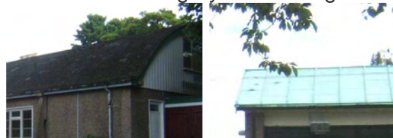
Non-traditional roofs at the churches of Longbenton conservation area
