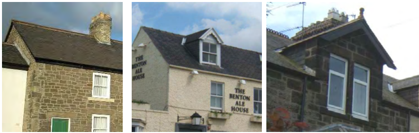
Dual pitched, un-hipped roofs prevail in Longbenton conservation area, but some do have dormer windows. Half dormers at Cheviot View
