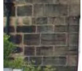
Rubble sandstone (Meth'ist Ch) and ashlar (M House)
