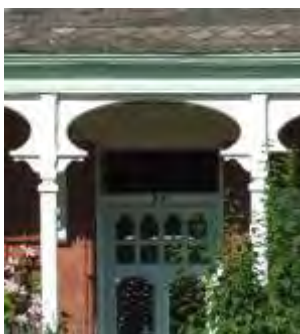
Typical doorway joinery, Suburban Growth Sub-Area
