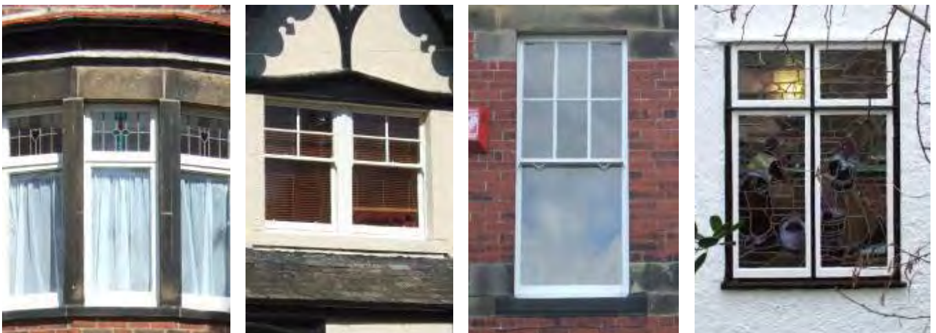
Typical Edwardian, 1920s and 1930s windows, Suburban Growth Sub-Area
