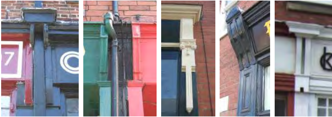
Shopfront brackets and mouldings are simple and elegant
