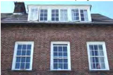
Neo-Georgian windows and typical Edwardian sliding sashes with smaller beaded top sashes
