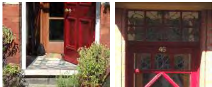
Lobby floor and overlight with timber beading, leading and painted glass
