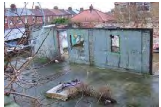
Derelict garage block and forecourt, Back Lane
