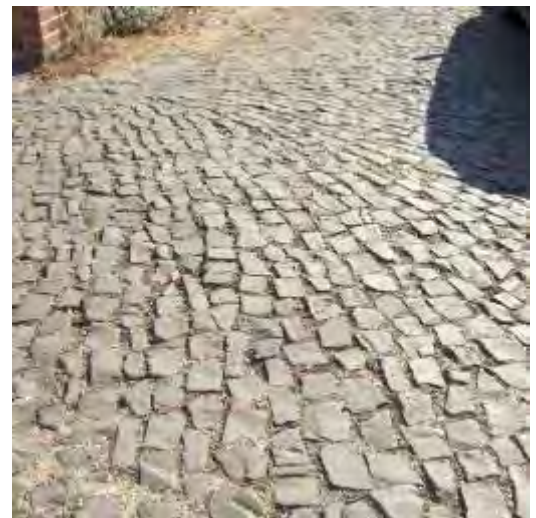
Historic kerbs, gullies, drive crossings & back lane surface
