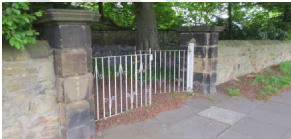
Figure 10: Grade II listed gate piers at Murton Farmhouse
