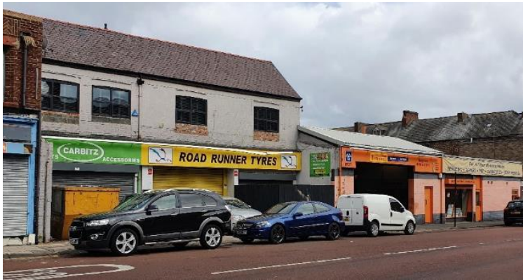
East side of Church Way
