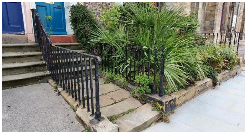
Surviving original railings and green garden
