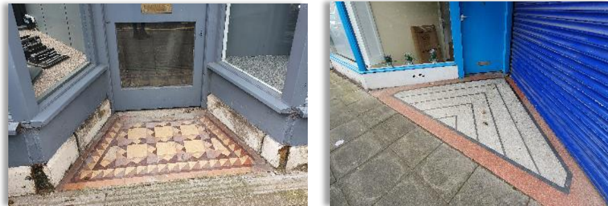
Traditional recessed doorways and decorative thresholds on Albion Road
