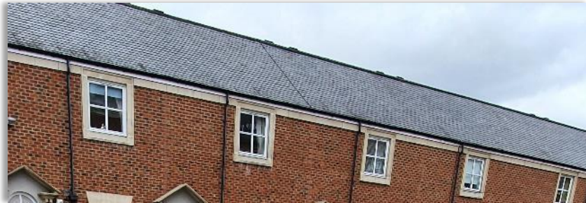
Chimneys are missed when they are not present
