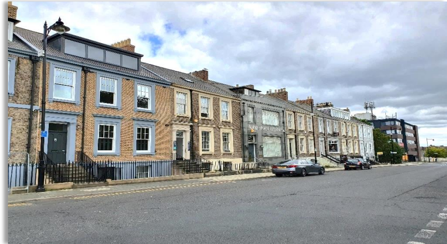
Three bay terraces with half-sunken basements on the east side of Northumberland Square
