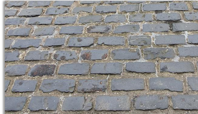
Reclaimed setts, southern part of Howard Street
