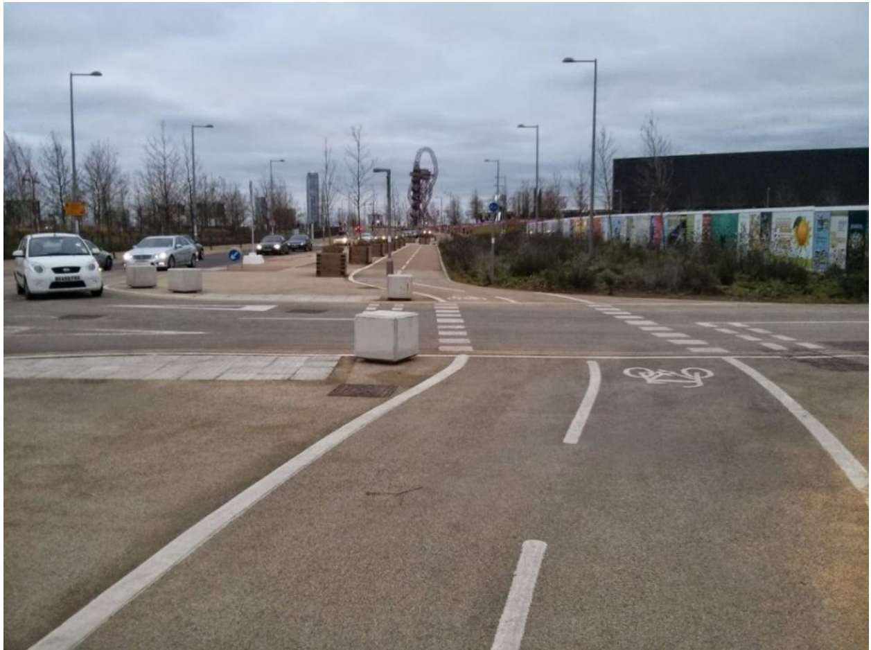
Figure C.2 – Example of continuous at grade side road treatment with vehicle giveways. Continuous at grade side road treatments encourage drivers to slow and take extra care at junctions giving way to pedestrians and cyclists providing continuous routes without a change in gradient;
