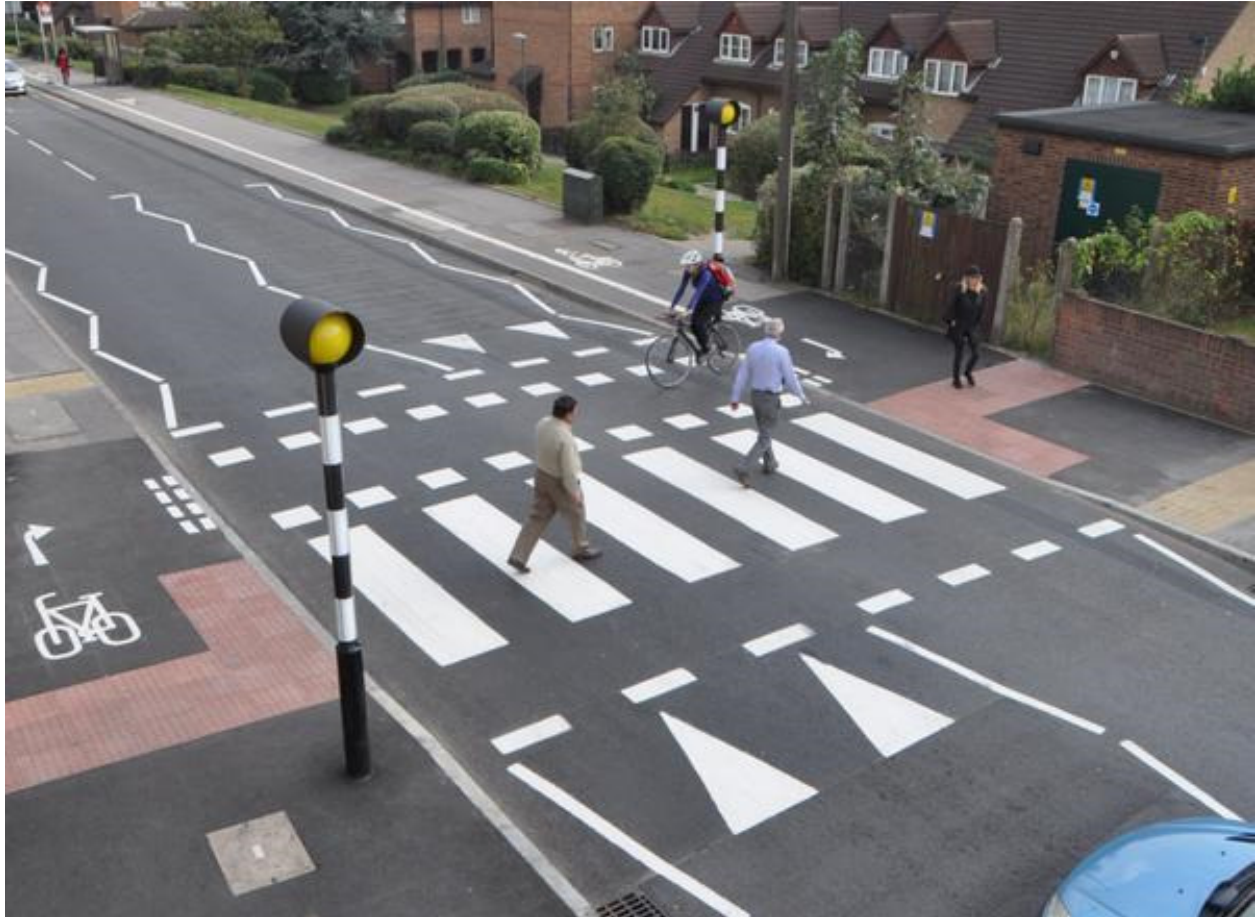
Figure C.4 - Parallel zebra crossings separate conflicting cycle and pedestrian movements allowing both pedestrians and mounted cyclists to cross the carriageway at the same time.
