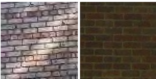
Mottled bricks in English garden wall bond, left, and darker bricks in stretcher bond, right
