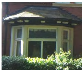
Angled stone sills and lintels at Lincluden
