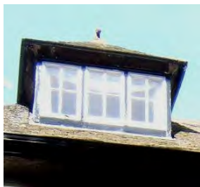
Dormer at Denham House
