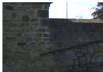
Stone rubble wall at Vicarage Cottage, above, and stone gate pier at the Old Vicarage
