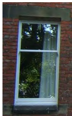
Angled stone sills and lintels at Lincluden
