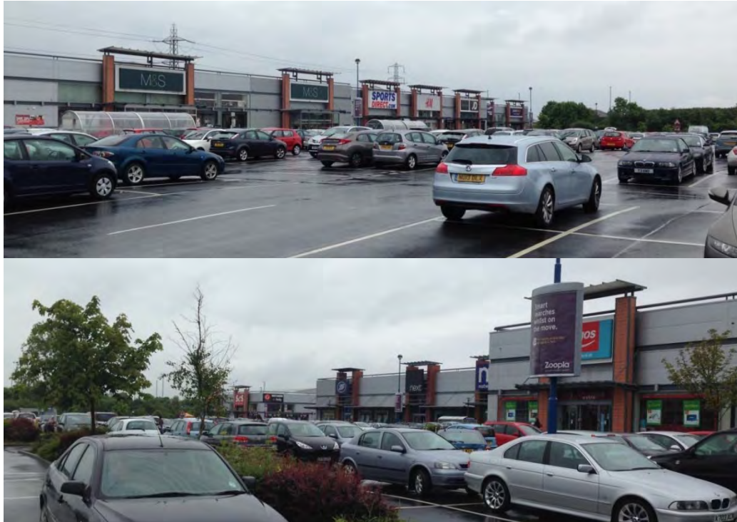
Figure 7.1 Silverlink Shopping Park, Coast Road, Wallsend
