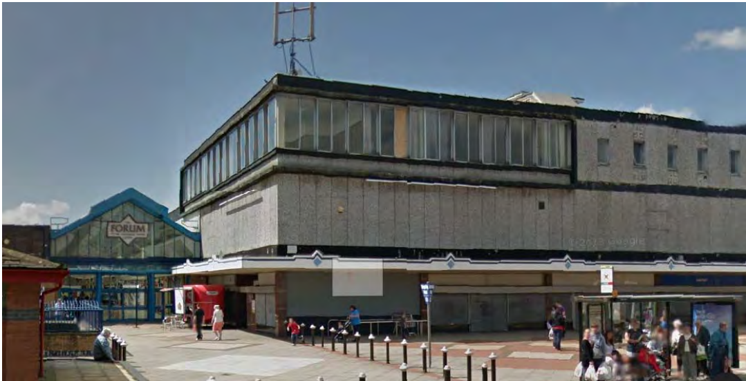
Figure 6.1 The Forum Shopping Centre, Wallsend (before & after refurbishment)
