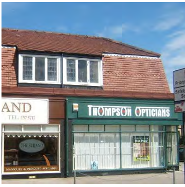
Mansard roof at Queensway
