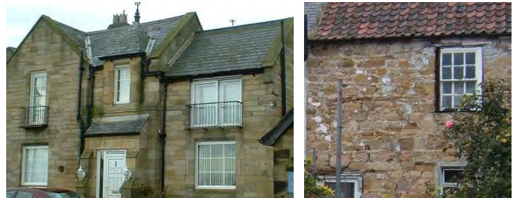
Ashlar 1 Old Coastguard Cottages and rubble 6 Well Close
