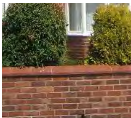
Typical wall in the Inter-war Semi-detached Properties Sub-Area
