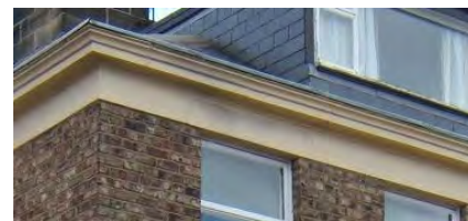
Stone verges on Northumberland Terrace
