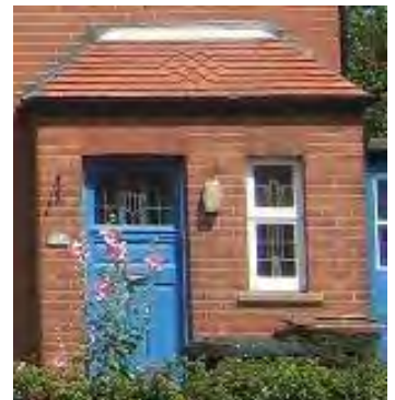
Brick porch on Queensway
