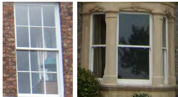
Original Georgian and Victorian windows
