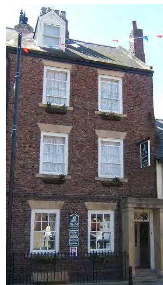
Typical Village Core building
