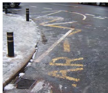
Duplicate road markings
