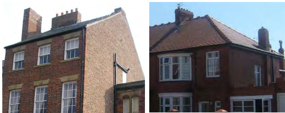
Unhipped and hipped roofs
