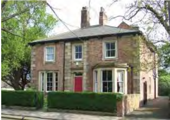
Detached, double-fronted, two storeys with pitch roof, The Villa
