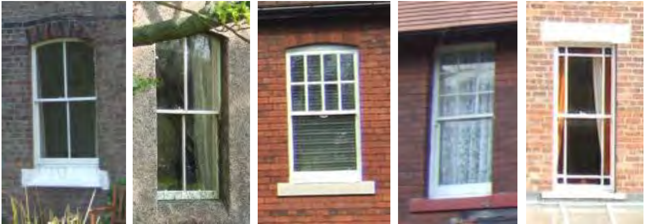
Victorian and Edwardian sliding sash windows, some with glazing bars only in the upper sash as decoration
