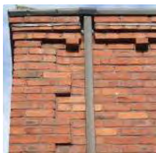
Brick detailing and coloured mortar, Whitehouse Mews
