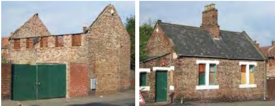
Burnt-out Coal House, Boyd Rd; Neighbouring Cross Hse Cottage may also have condition or vacancy issues
