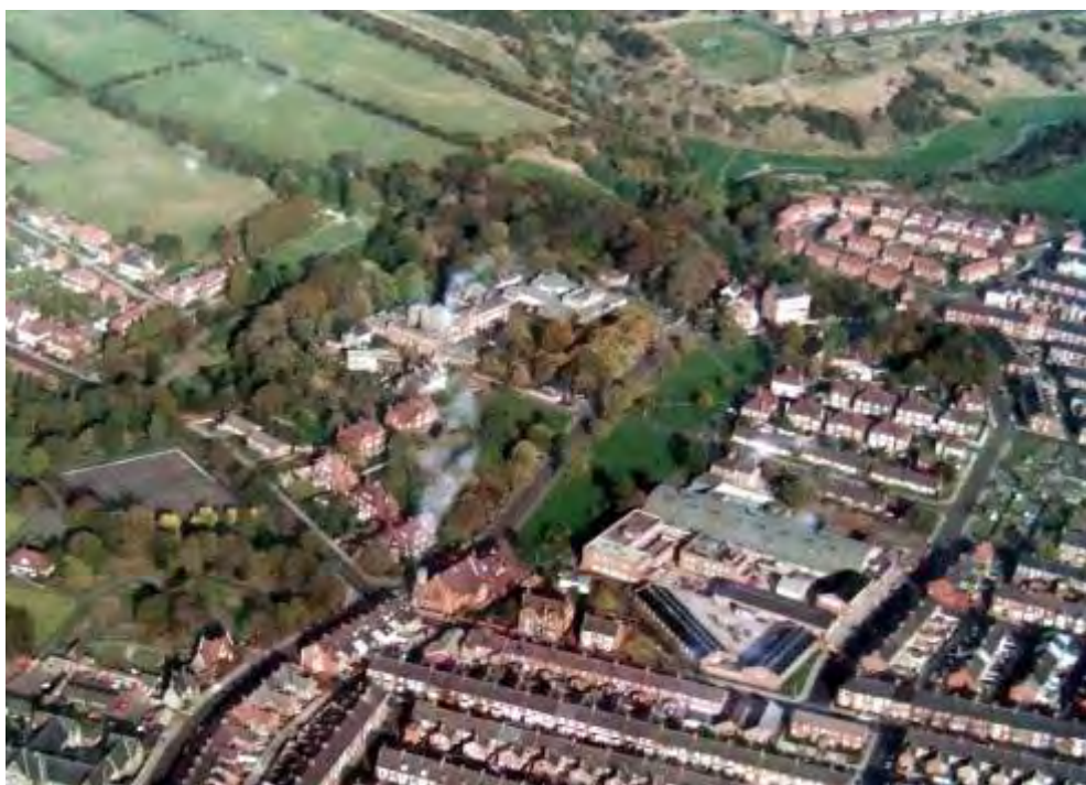
Oblique aerial photograph from the south-west, c.1980s. Note the former ice rink and large commercial buildings
