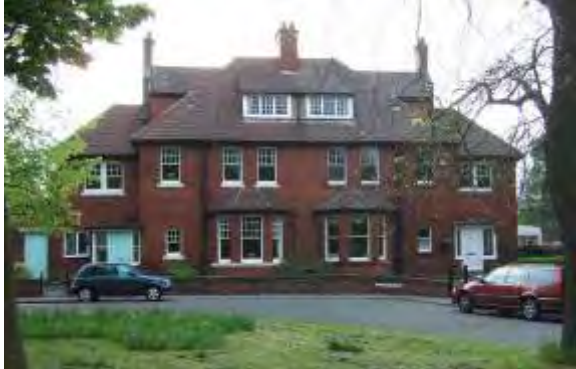
Two storey semis with attic space and stepped wings, Park Villas
