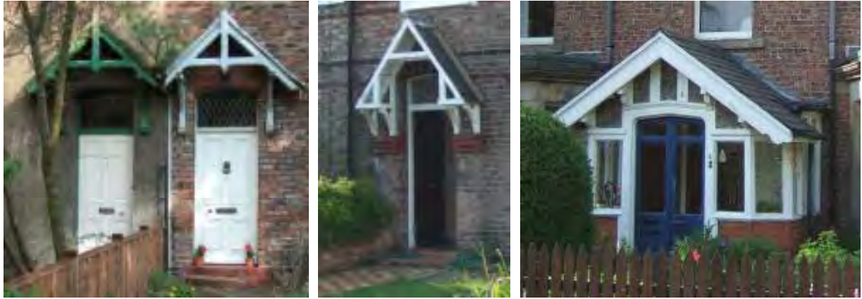
Above: Victorian doorways with timber hoods on brackets, and an ornate half-glazed porch (East and West Vilas, Elm Terrace)
