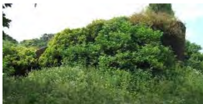
Overgrown Vinery walls, Hall Grounds
