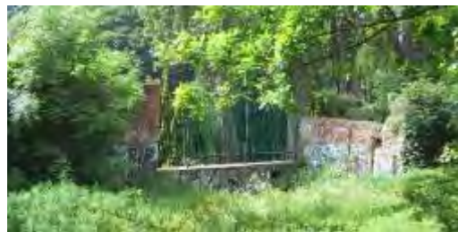
Important but ruinous viney walls and other structures
