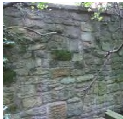
Rebuilt local sandstone boundary wall, The Villa
