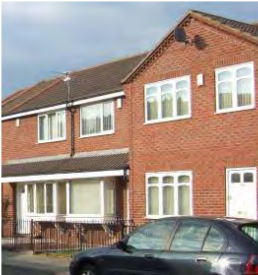
Windows in the South Sub-Area
