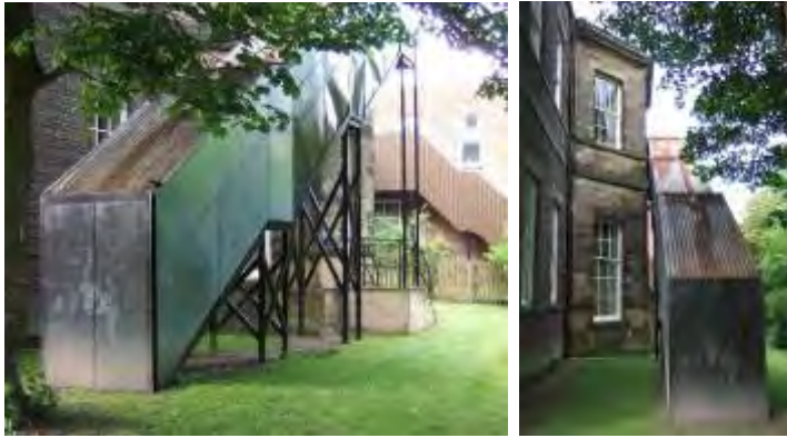
Ugly fire escapes to the rear of the Hall block notional views across its Grounds
