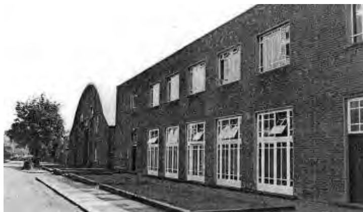
The former skating rink (left) and DSS offices (originally a Daimler car showroom), demolished in the late 1980s
