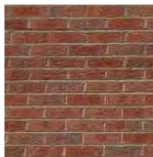
Modern brickwork in stretcher bond, South Sub-Area
