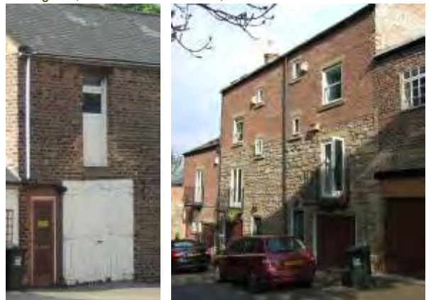
Functional openings at former brewery, some now modernised
