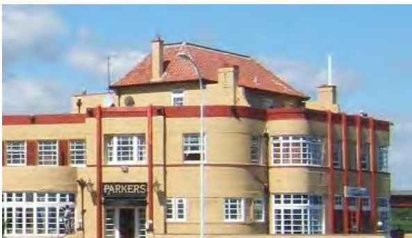
Unusual roofscape at the Park Hotel
