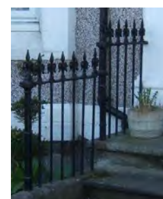
Rare surviving railings
