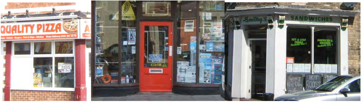
Retention of features: finials and pilasters, left, and curved recessed doorway, right. Good retention of original features at Smithy's
