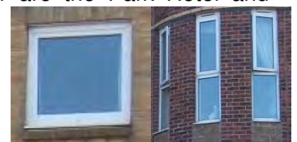
Differences in windows within the conservation area's more modern developments
