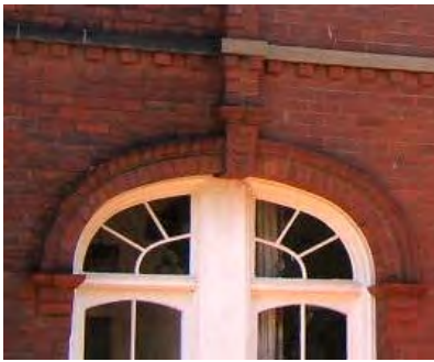
Brick detailing at 30 and 32 Beverley Gardens
