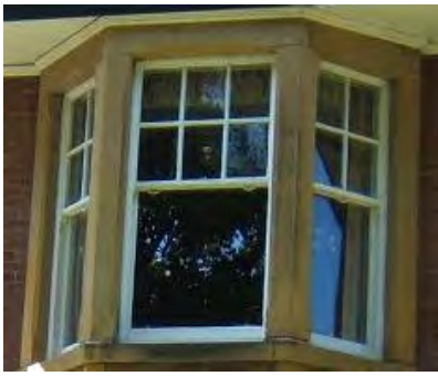
Glazing bars used in the top sash on Beverley Gardens
