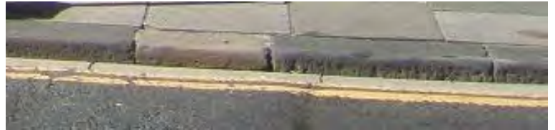
Granite kerb on John Street
