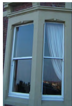
Original Victorian windows at Beverley Terrace
