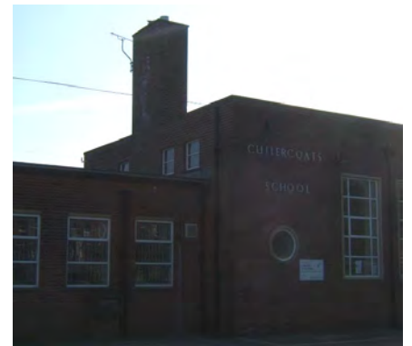
Flat roof at Cullercoats Primary School
