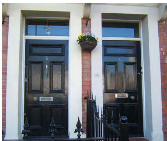
Good original doors at 6 and 8 John Street
