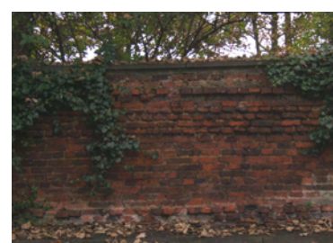
Brick wall at Castles Green
