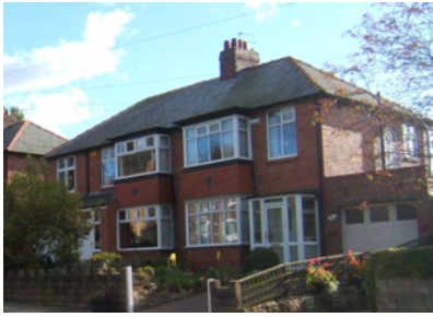
Loss of symmetry caused by over-garage extensions
