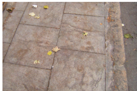
Stone pavement and granite kerbs
