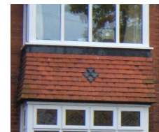
Red clay tile hanging at 1 Hillside
