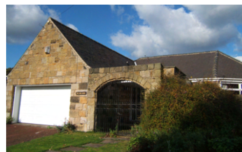
Mill House, a one-storey property with retention of agricultural character
