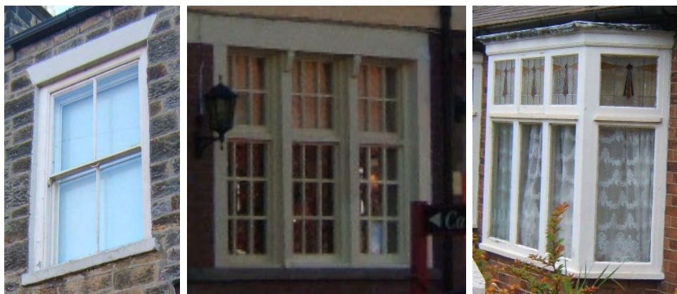
Sliding sash windows, and later examples with decorative glazing bars. Plus, casements with painted glass
