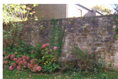
Stone wall at Killingworth Park
