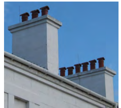
Chimneys are tall and intact
