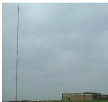
Transmission station and mast
