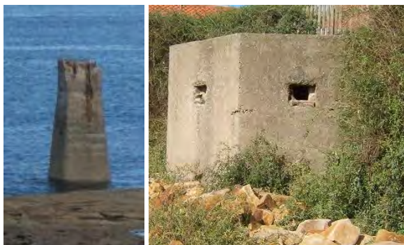
Military remnants: concrete pillar (left) and pillbox (right)
