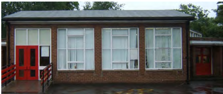
Original doors and windows
