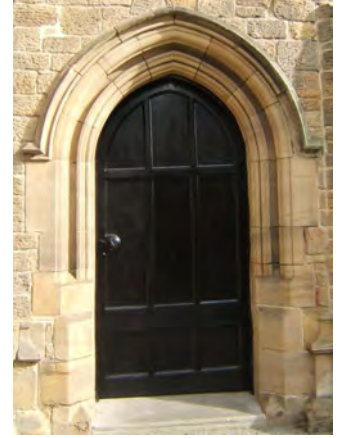
Timber door in stone surround
