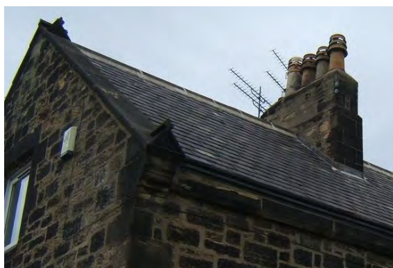
Roofs and chimney at Cemetery Lodge
