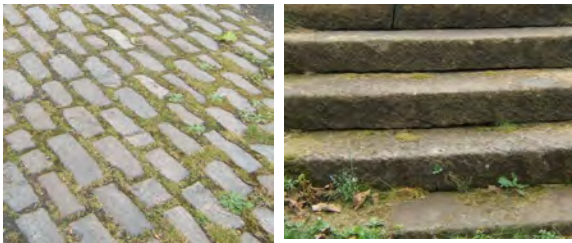
Granite setts and steps in Church Bank Cemetery
